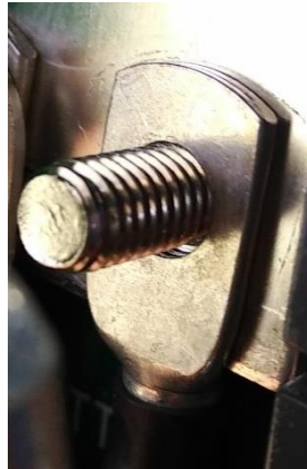
Figure 9: Close-up view GND bolt with inside out ring cable lug
