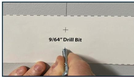
2. Mark all six holes by pressing the tip of a lag screw through the center of each cross mark.
