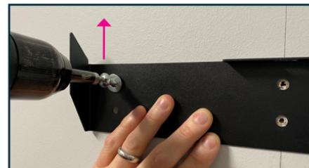
6. Hand screw in bolts into the zip toggles. Use drill to tighten down.
