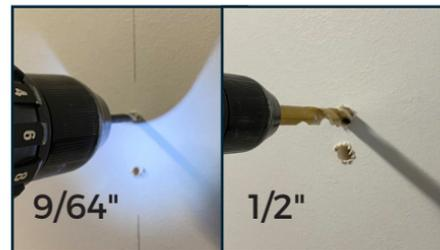
3. Using a 9/64" drill bit, drill two pilot holes for the lag screws. Using a 1/2" drill bit, drill four holes for the zip toggles.
