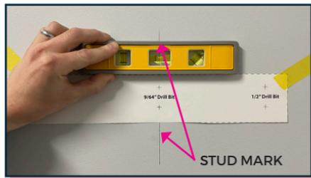
1. Locate stud within the wall you intend to hang your Reflect and mark with a pencil. Level and tape wall mount template with middle two cross marks centered over stud mark.
