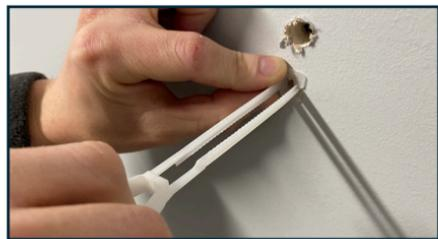
4. Insert zip toggles into 1/2" holes and push the zip toggle plate until it is flush against the wall.
