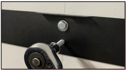
7. Drive in the two lag screws into the pre-drilled pilot holes.
