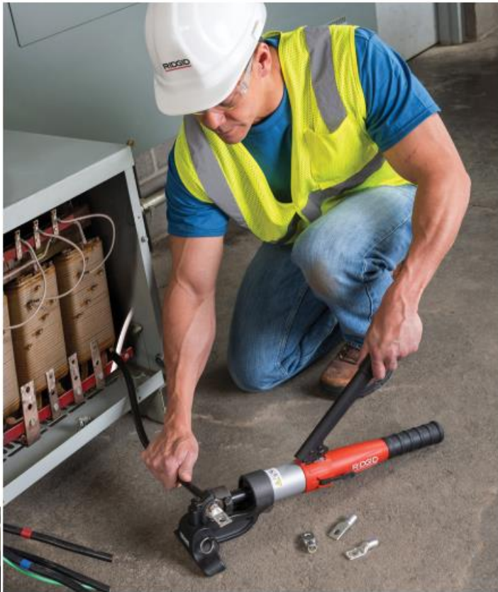
Courtesy of RIDGID®. RIDGID® is the registered trademark of RIDGID, Inc. Figure 3-9. Using a hydraulic crimper to attach a lug to the end of a large conductor.
