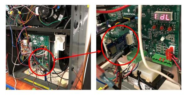
To load Shared Data onto a **ComfortBridge**<sup>™</sup> unit, first insert the card into the Shared Data programming connector on the control board inside the desired **ComfortBridge** unit. Then ensure the board and the card are receiving power. Once the board is fully powered on and displaying the "IdL" code, use the "LEFT", "RIGHT", and "CENTER" buttons on the control board to navigate the appropriate menus on the control board.
