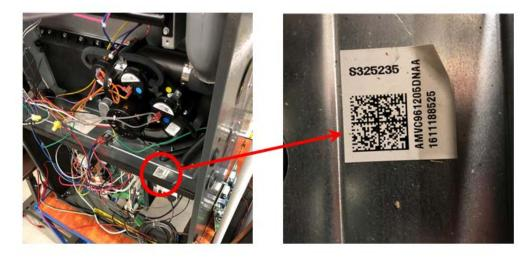
For this **ComfortNet**<sup>™</sup> furnace, the 2D barcode is located on the blower deck, its model number is AMVC961205DNAA
