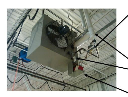
Condensate Pumped Into Flex Hose Up to Ceiling & Pitched Down to Nearest Floor Drain Across Room
