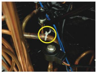
9. With using a slot screwdriver, lift up the on the side tab to pry the cover off from the RTV. Be sure not to break the tab.
