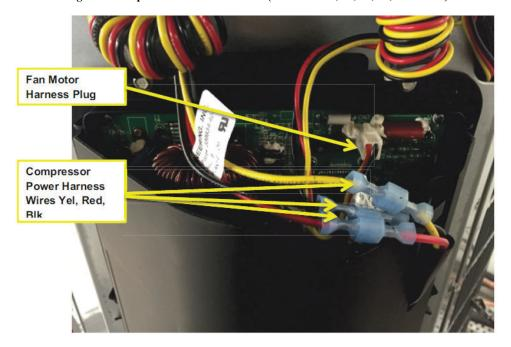
Fig. 33 – Compressor and Fan Harness (Unit size 24)
