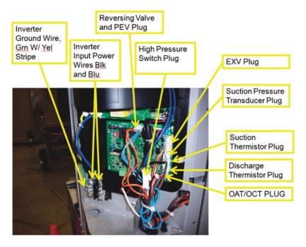
Fig. 34 – Wire Harness Connections (Unit sizes 25, 36, 37, 48, 49 and 60)
