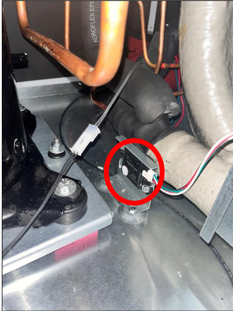
RDS Sensor in YT Compressor Section
