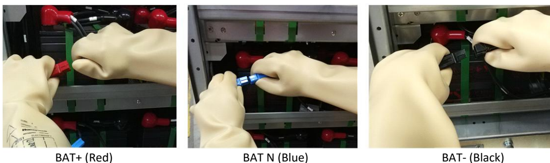
Figure 3-2 Connecting battery internal terminals
